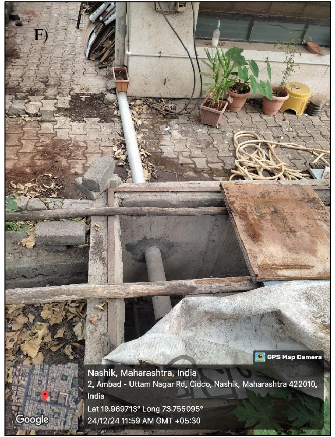
Figure E) & F) Inlet of the rainwater to the storage tank
