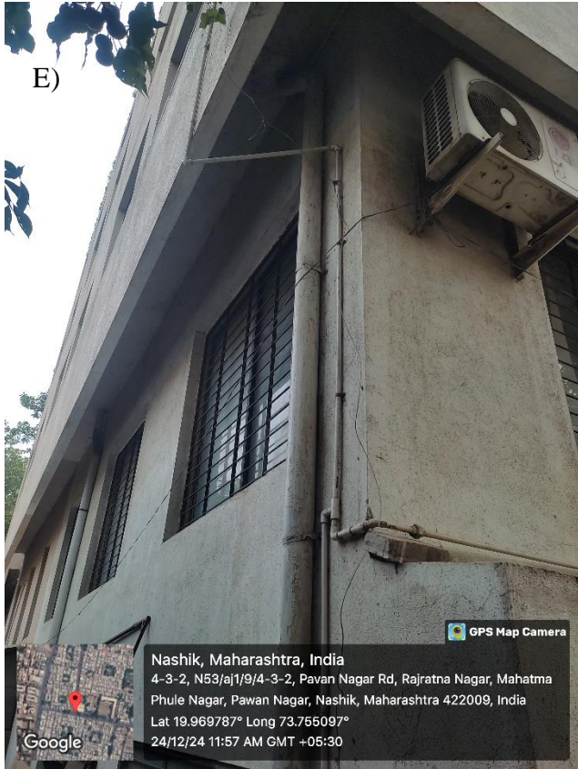
Figure E) & F) Inlet of the rainwater to the storage tank
