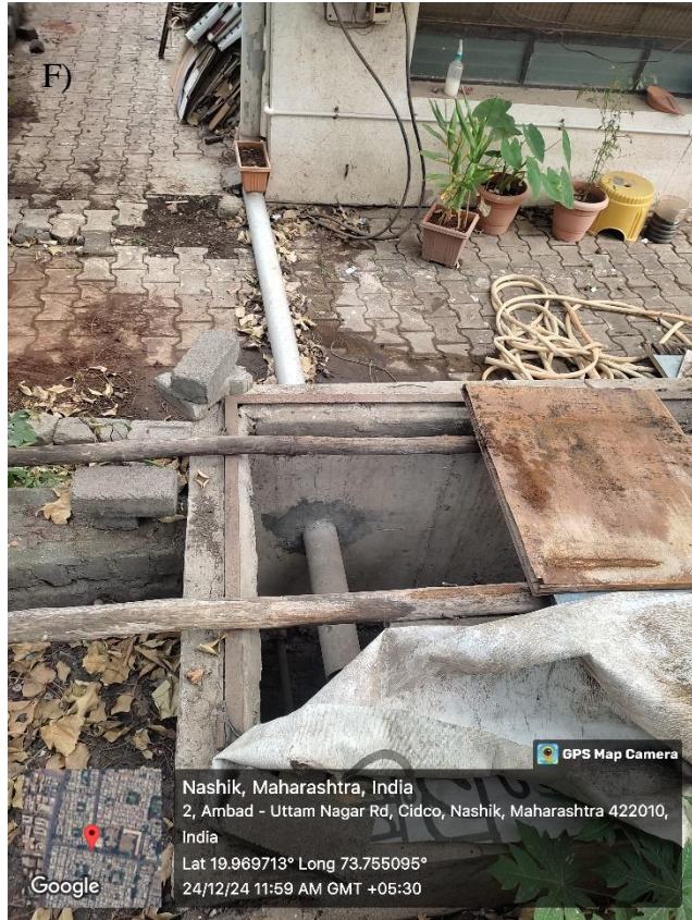
Figure E) & F) Inlet of the rainwater to the storage tank
